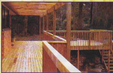
**FACT 4** Outdoor timber structures must be correctly fixed or fastened on to timber frames at the correct spacing to avoid likely twisting, cupping, or other distortion causing damage and loss. The structure must also be appropriately maintained.
