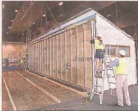
Home and away: Prebuilt Housing Solutions' revolutionary home can be folded up and delivered on the back of a truck.
