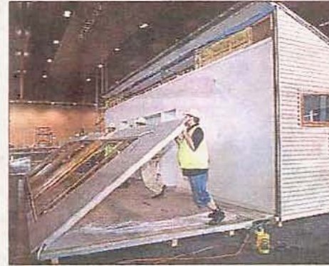
Home and away: Prebuilt Housing Solutions' revolutionary home can be folded up and delivered on the back of a truck.
