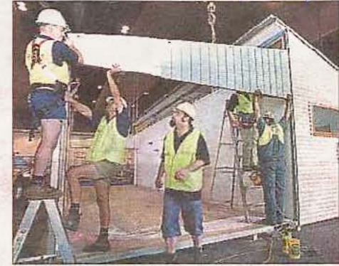
Home and away: Prebuilt Housing Solutions' revolutionary home can be folded up and delivered on the back of a truck.
